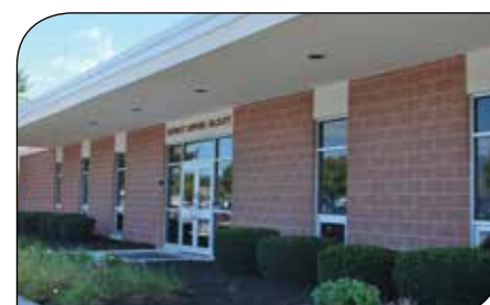
District Office/District Support Facility 6746 Carlisle Pike Mechanicsburg, PA 17050 Phone: 717-697-8261
