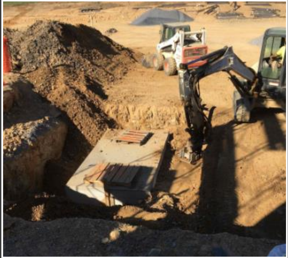
Grease interceptor for Kitchen area installed
