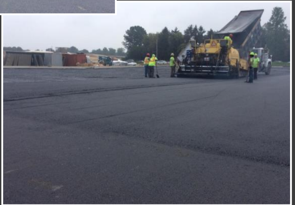
Placed base course of asphalt in the elementary school parking area
