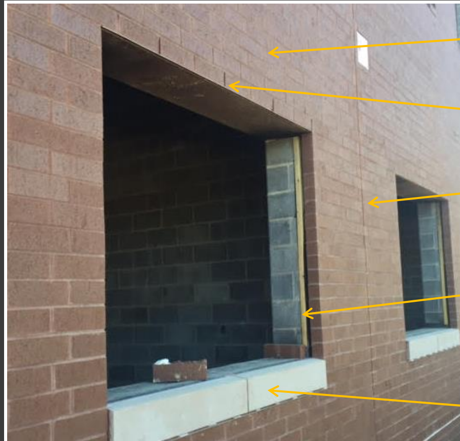
Installation of the exterior brick veneer and the precast concrete window sills in Area A
