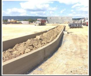
Start of the concrete curb and subbase in the parking area
