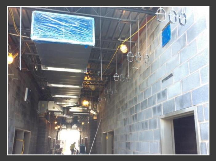
Mechanical ceiling rough-ins have started with Area A-East 1<sup>st</sup> floor corridor ductwork.
