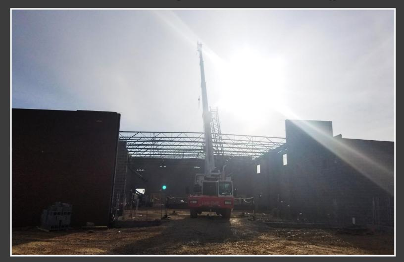
Lobar subcontractor began installing the long span roof steel for the gymnasium and stage area
