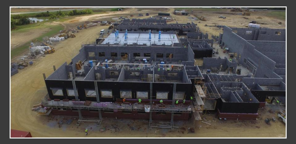
Lobar subcontractor is continuing laying the face brick on the North building elevation
