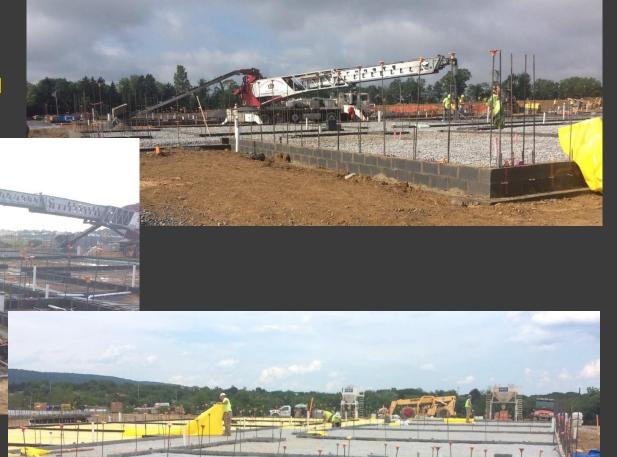
05/31/17 – Lobar installed vapor barrier in Area B1
