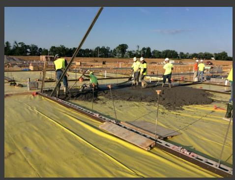
06/02/17 – Lobar placed the concrete slab on grade in the North classrooms of Area B1
