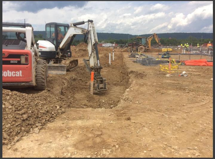
05/31/17 – Silvertip subcontractor backfill of underground sanitary piping main down through corridor B123
