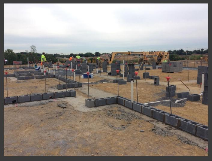
05/26/17 – Lobar subcontractor installed CMU foundation walls in Area B2
