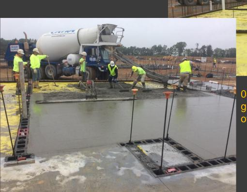
05/30/17 – Lobar placed the concrete slab on grade in the South classrooms and stairwell of Area A-East
