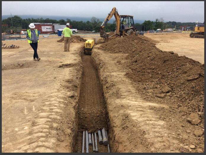
05/22/17 – Boro continued install of underground feeder conduit from Area A Electric Room towards main electrical room in Area C
