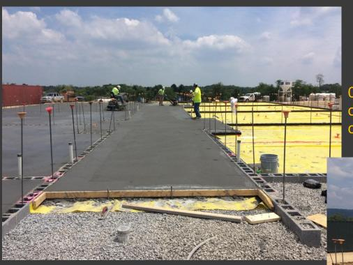
05/24/17 – Lobar finished the concrete slab on grade in the North classrooms and wing corridor of Area A-East
