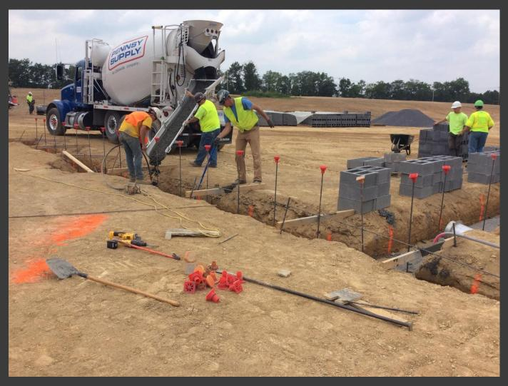
05/24/17 – Lobar placing concrete footers in Area C1
