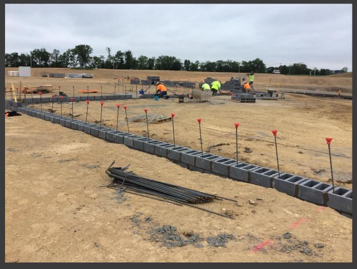
05/22/17 – Lobar subcontractor placing perimeter CMU foundation walls in Area C2
