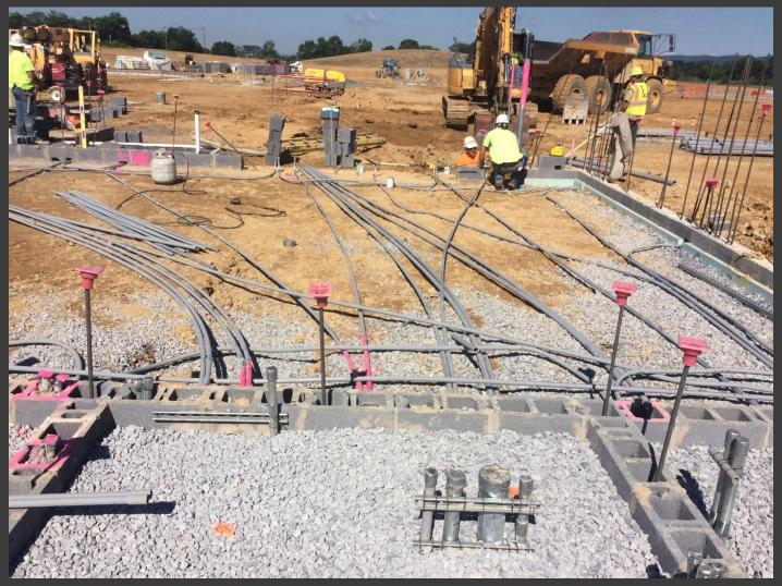
06/01/17 – Boro installing underground feeder conduit from Area B2 to main electrical room in Area C
