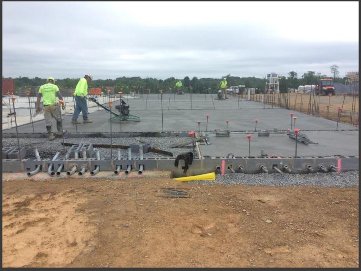
05/30/17 – Lobar finished the concrete slab on grade in the South classrooms and stairwell of Area A-East
