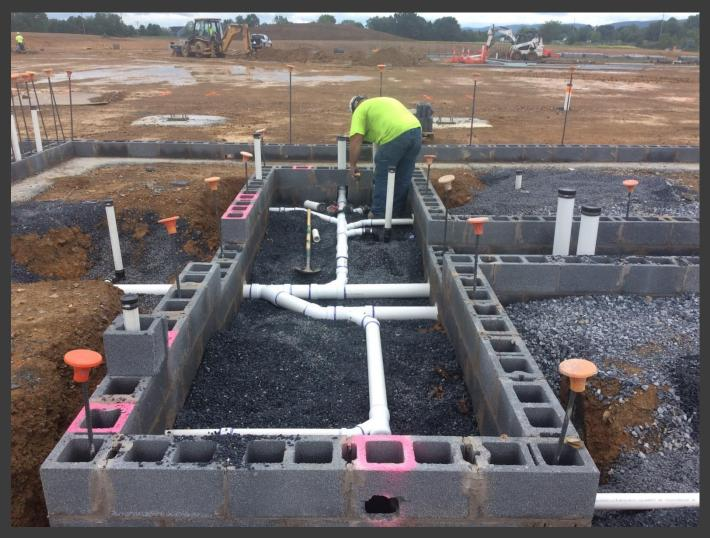
05/26/17 – Silvertip installed underground sanitary piping in Area B1 restroom pipe chase
