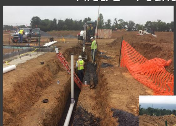
05/30/17 – Silvertip continued install of underground sanitary piping main down through corridor B123
